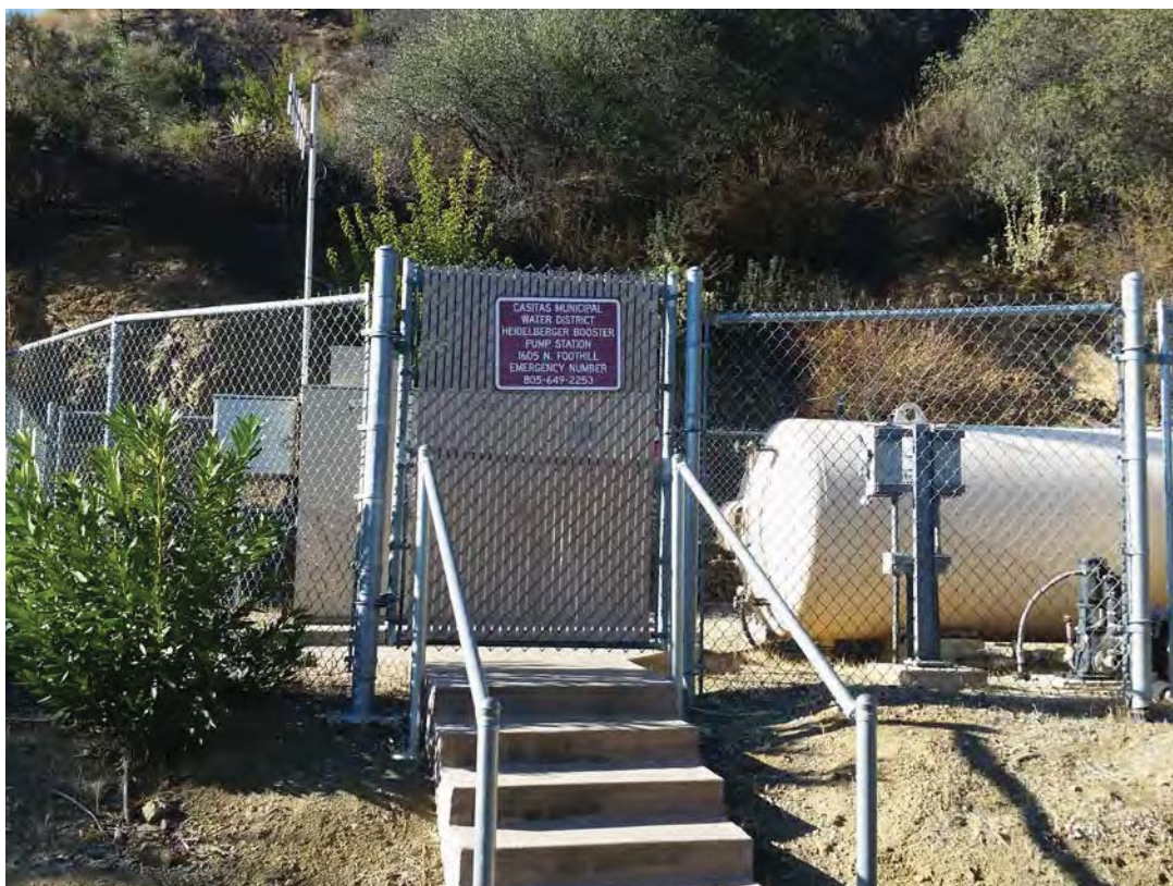
Photo 2. Heidelberg Booster Pump Station, facing west
