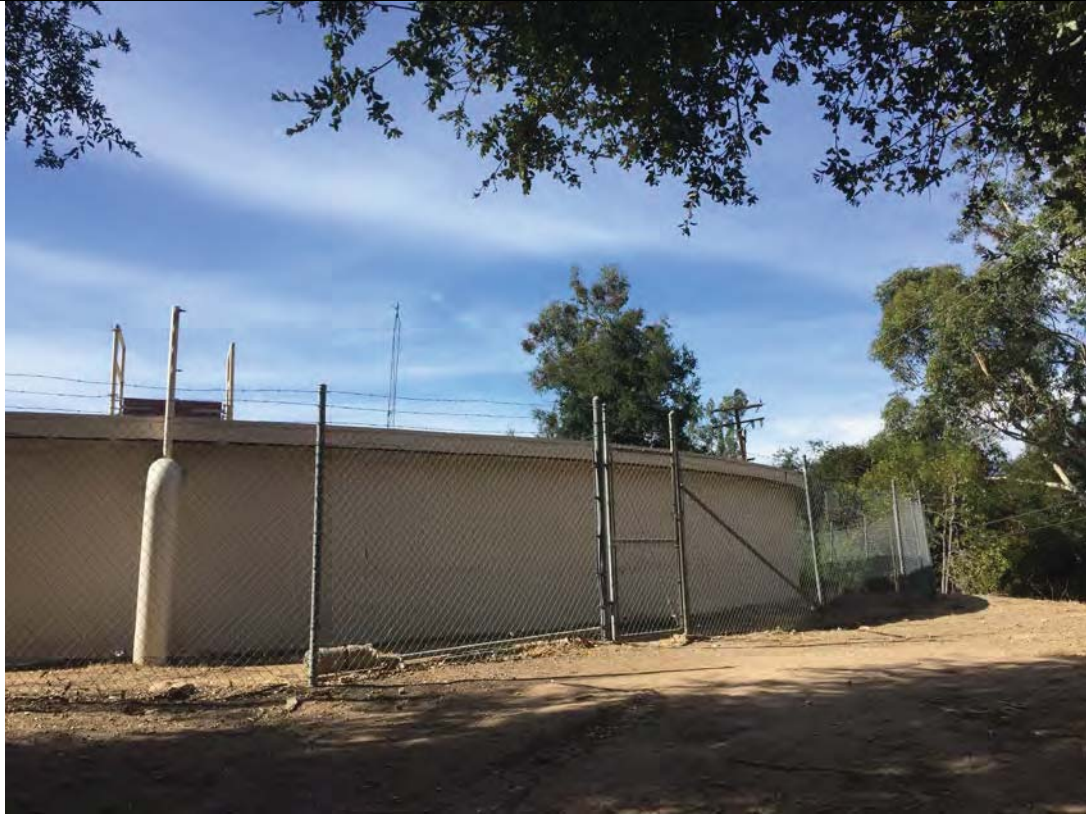
Photo 7. W Arbolada Tank, facing southwest
